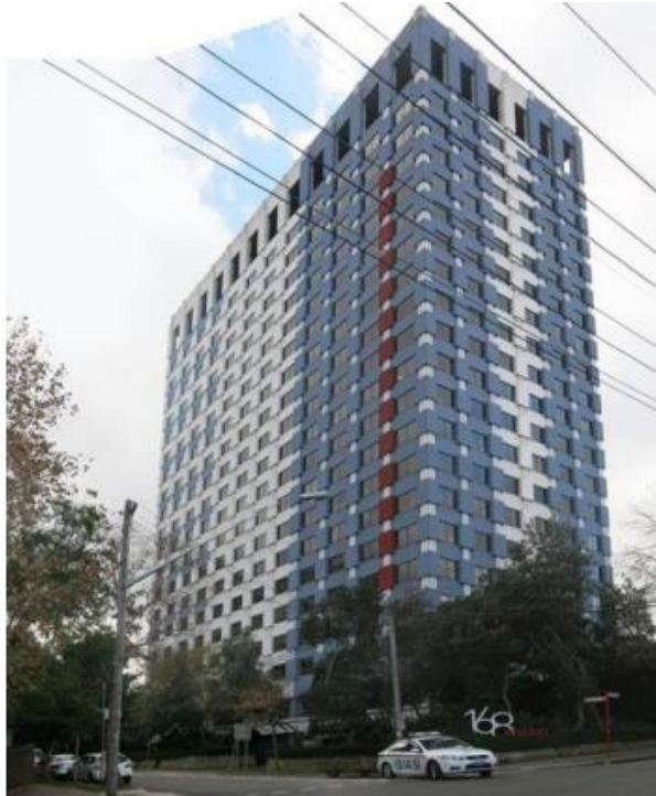
Existing Office Building
